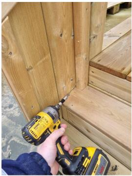
3. Place the ramp into position as shown. Fix the ramp to the tower using  $4 \times 100$ mm screws through the pre-drilled holes (2 screws per side)
